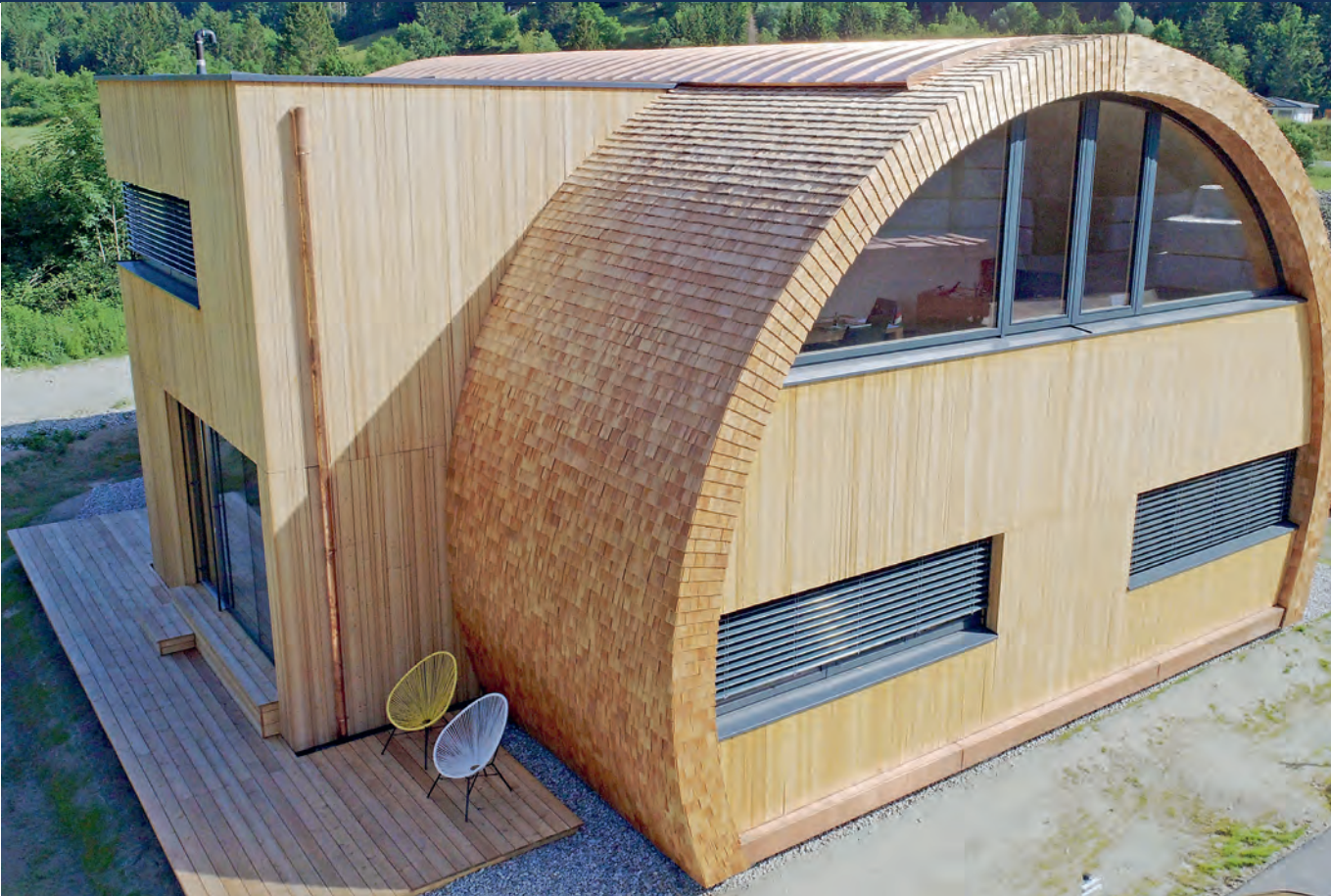
An example of modern timber construction combined with tradition (shingle roof).
