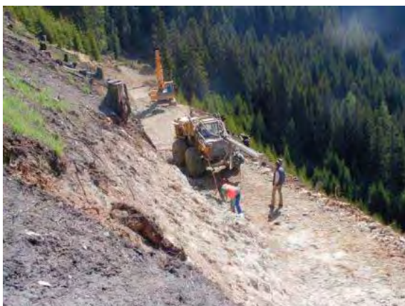
Picture 16: Preparation for Blasting
