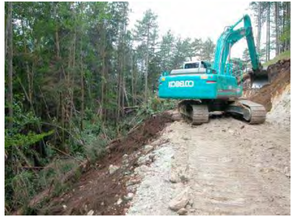
Picture 7: Excavator deposits topsoil directly into the final position on the fill side
