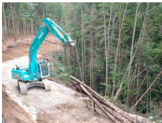
Picture 3: Log removal by excavator and storage alongside the road
