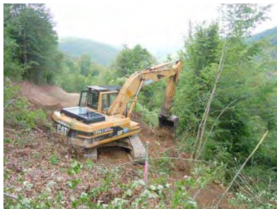
Picture 5: Remove the humus soil layer from the construction area. Covering the completed fill side with the humus soil
