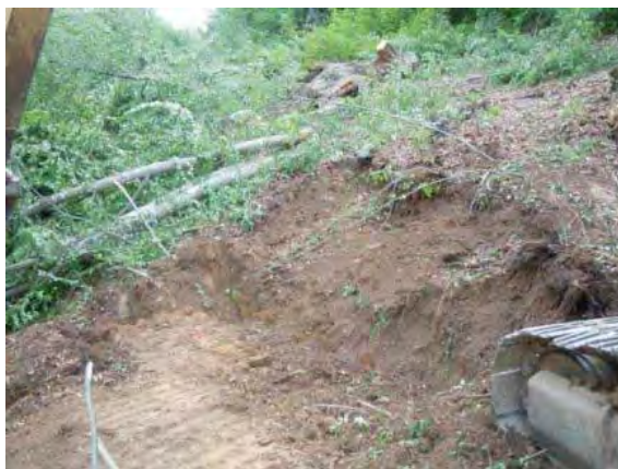
Picture 9: Forming the foundation for the forest road
