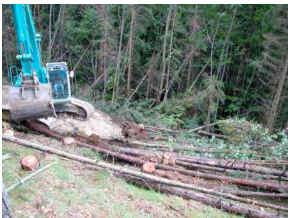
Picture 3: Log removal by excavator and storage alongside the road
