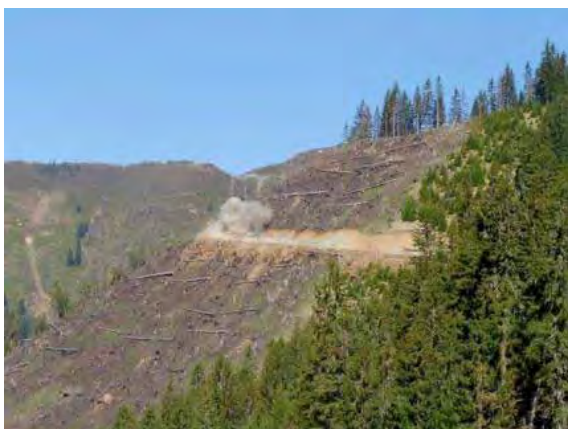
Picture 17: Blasting on forest road constructing site
