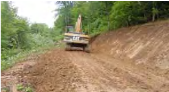
Picture 13: Preparation of the of the cut side in the right angle and arranging of the final layer of the subgrade without extra gravel
