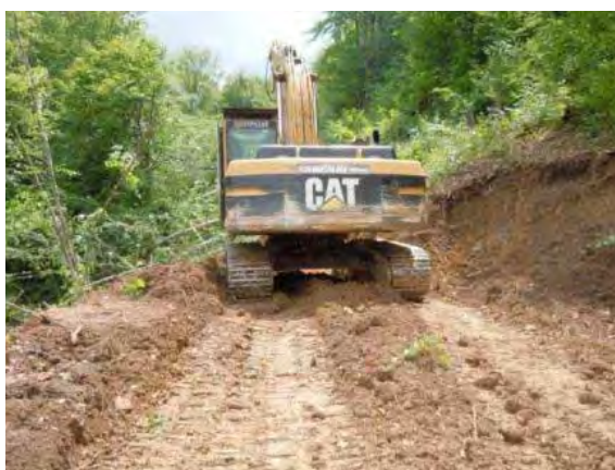
Picture 12: Continuous compaction of the layers by the tracks of the excavator or compactor (Hagauer, D. and Zöschner, H.: 2013; Best Practice Guidelines, Forest Road Planning and Construction, Adaptive Sustainable Forestry Management in Borjomi, Georgia)
