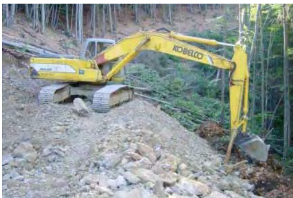
Picture 8: Excavator arranging the topsoil in correct positional arrangement
