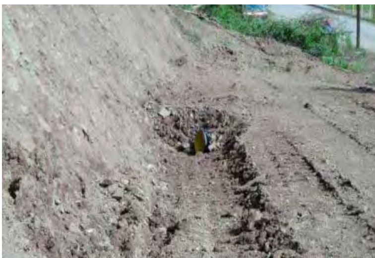
Picture 20: Intake of a culvert (not reinforced)
