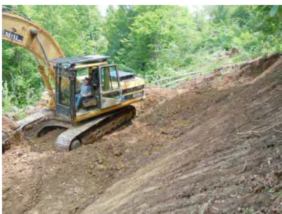
Picture 11: Building up the fill in layers with the material coming from the cutting side
