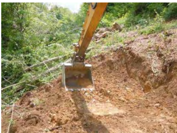
Picture 10: Compacting the foundation very well with the bucket of the excavator
