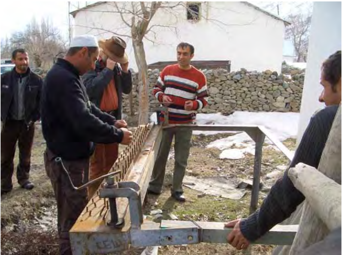
Gabion Construction close to Khorog, Tajikistan (Foto: B. Neussel)
